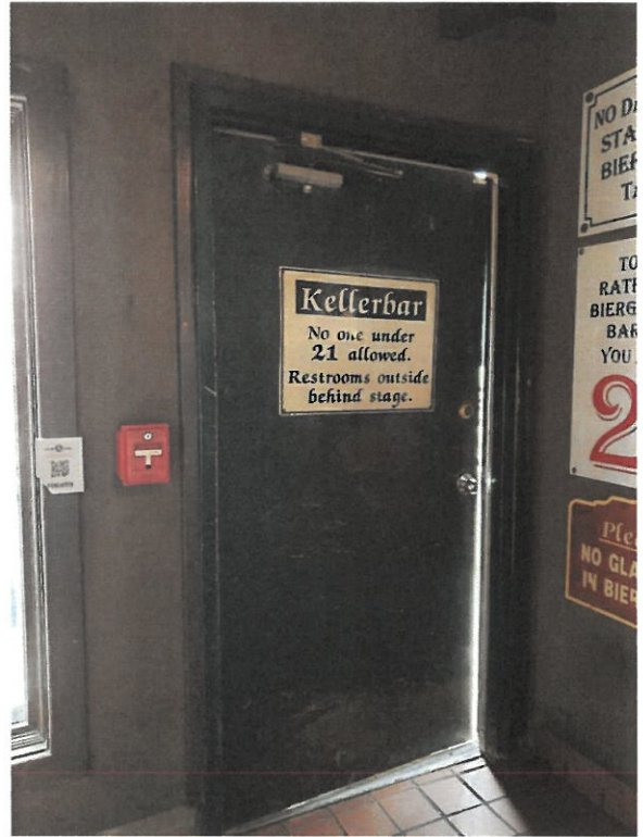
Fire alarm; Rathskeller door between indoor bar and biergarten
