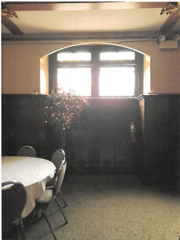
Fire extinguisher; Basement level, west wall in the Grand Kellersal
