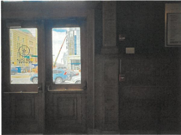
Fire alarm; Inside main entrance to first floor vestibule
