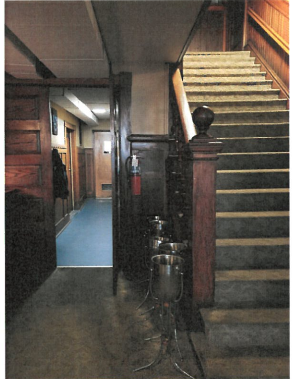
Fire extinguisher; Basement level, outside hallway to men's restroom in Rathskeller dining room
