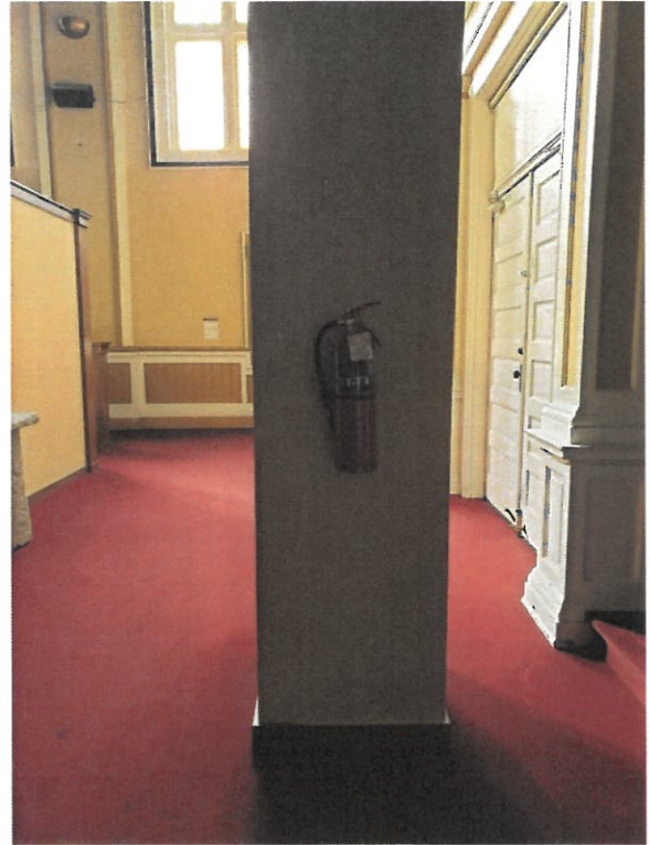
Fire extinguisher; Back of theatre, mounted to pillar between doors
