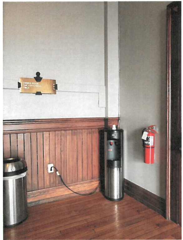
Fire extinguisher; Second floor landing outside YMCA offices and classrooms
